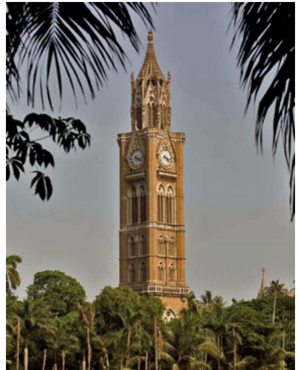
Rajabai clock tower, University of Mumbai, Fort Campus
